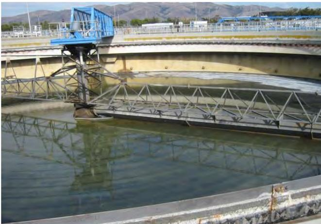
Figure 2— Picture of Clarifier interior and mechanism
