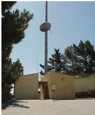
Caldwallder Reservoir Radio Tower
